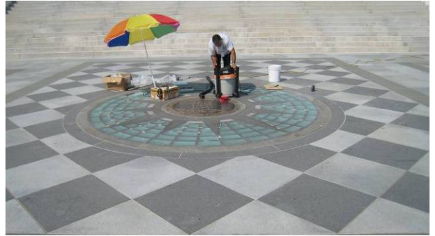
The oculus brings daylight into the rotunda space below through glass blocks, centered on the bronze seal of the Commonwealth in a compass orientation
